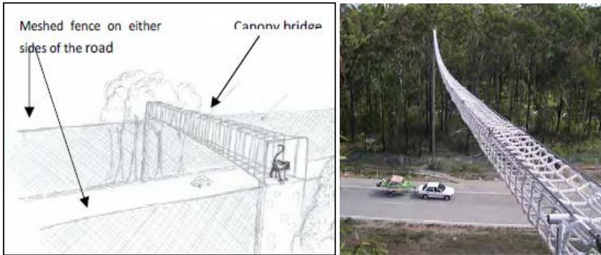
**Figure 5.2: Examples of canopy bridge designs**
